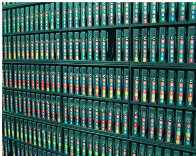
Data Center – Prodeb
